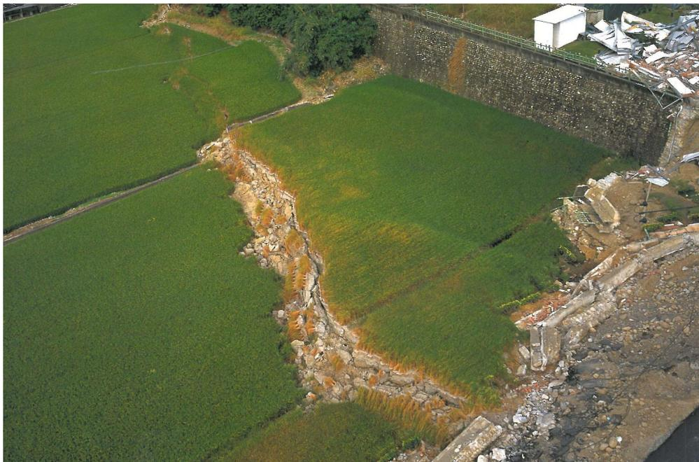
Figure 6. A retaining wall in the Quanjiafu Community collapsed during the 921 Jiji earthquake in 1999 (Lian, 1999).
