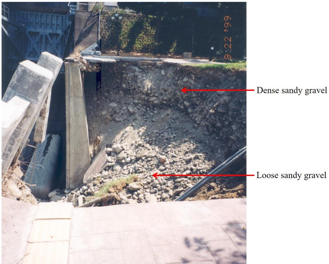
(a) Different states of sandy gravel on both sides of the failure surface.
