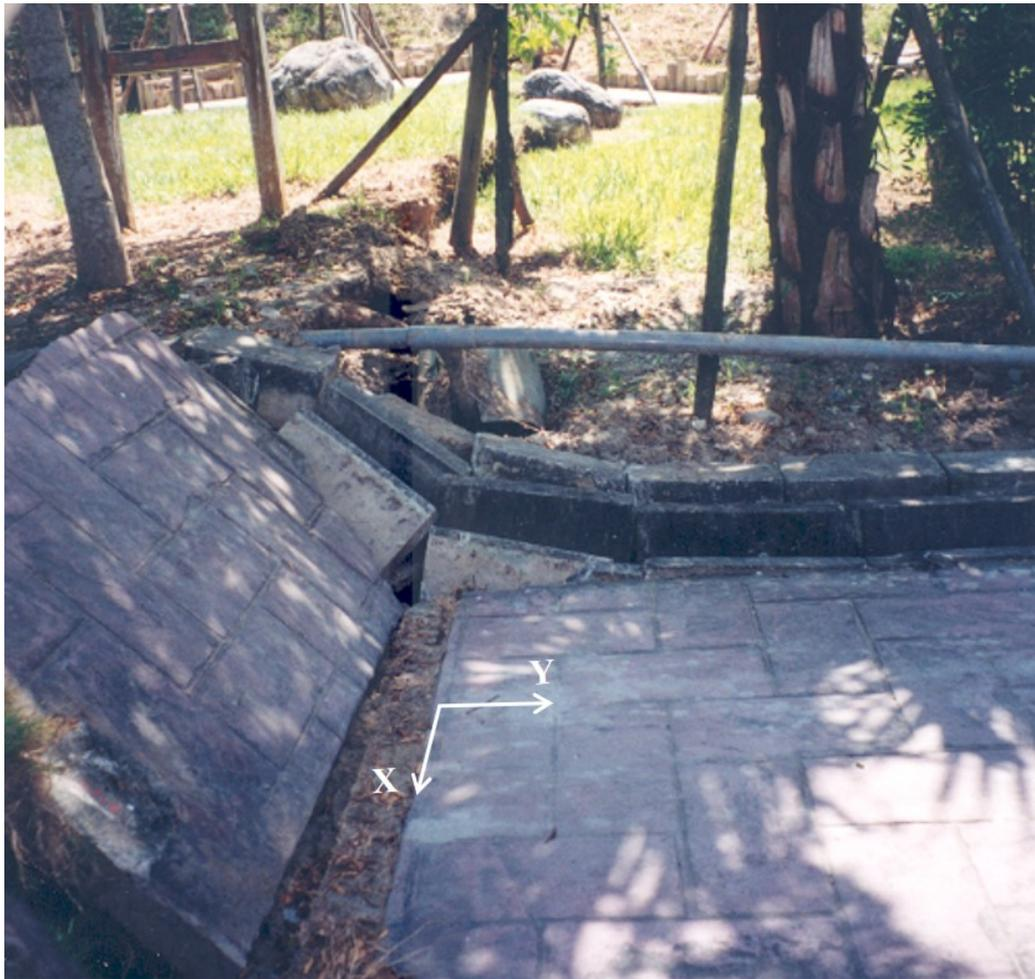
(b) Bidirectional shear-band tilting effect on the soil behind the collapsed retaining wall
