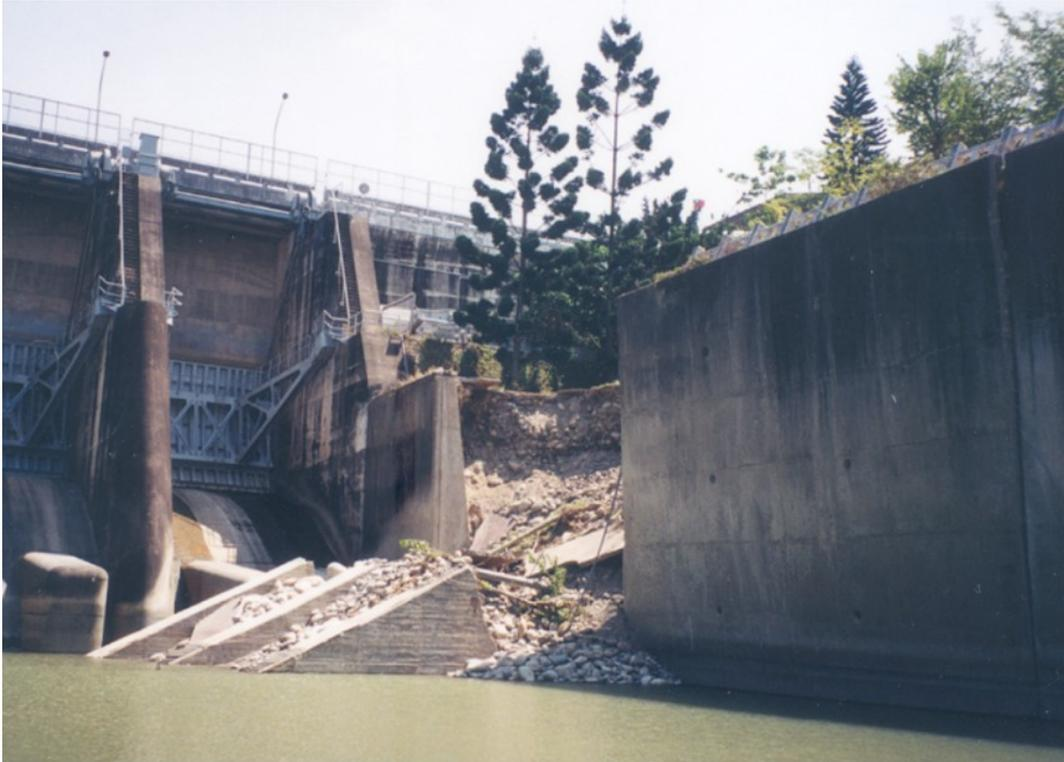
(b) Separated sandy gravel and retaining wall slipped to the riverbed.
