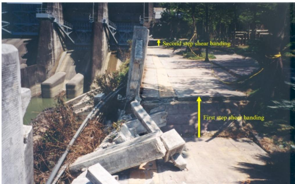
Figure 8. Local collapse of a shear-band retaining wall on a riverbank (right bank of the downstream Shigang Dam in Taiwan).
