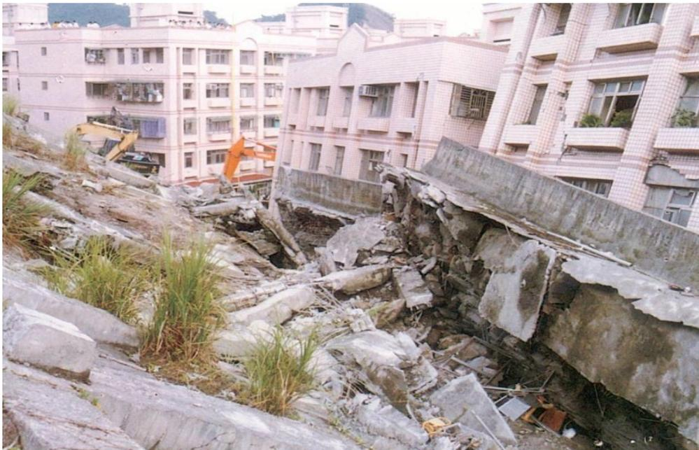
Figure 5. A retaining wall in Lincoln County collapsed in heavy rain (New Taipei City Government, Taiwan, 1997).
